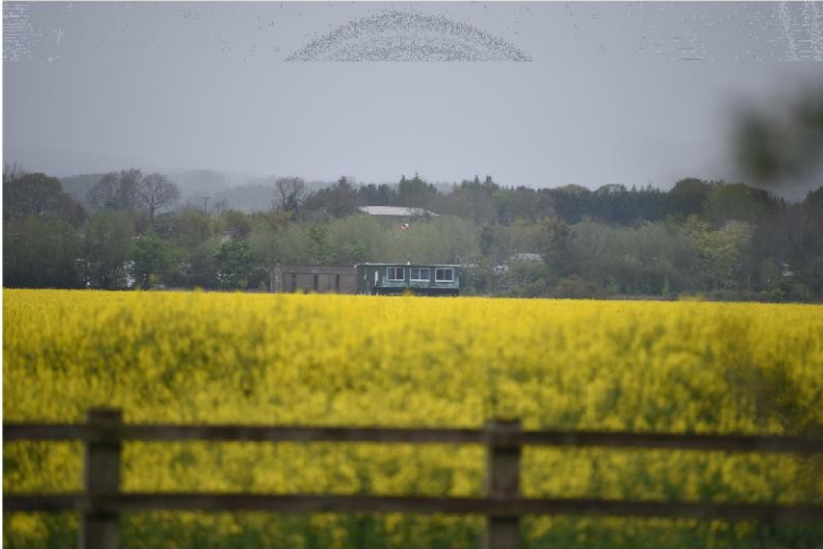
Wombleton Control Tower
