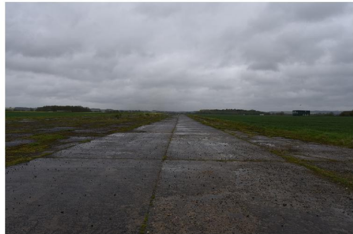
View towards Runway 04/22 from 35 end
