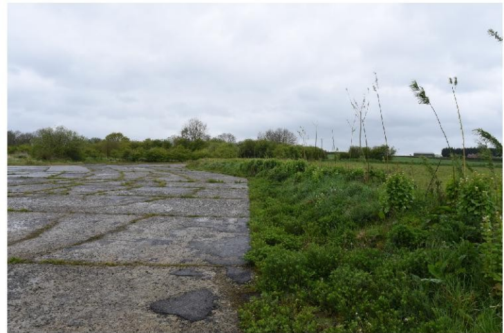
Runway 17/35 end bund
