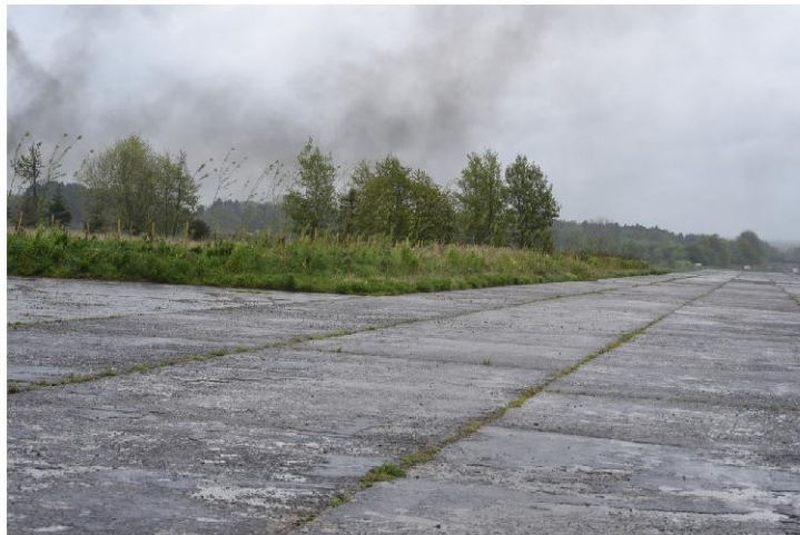
Opposite side to Runway 17/35 looking south (bund)
