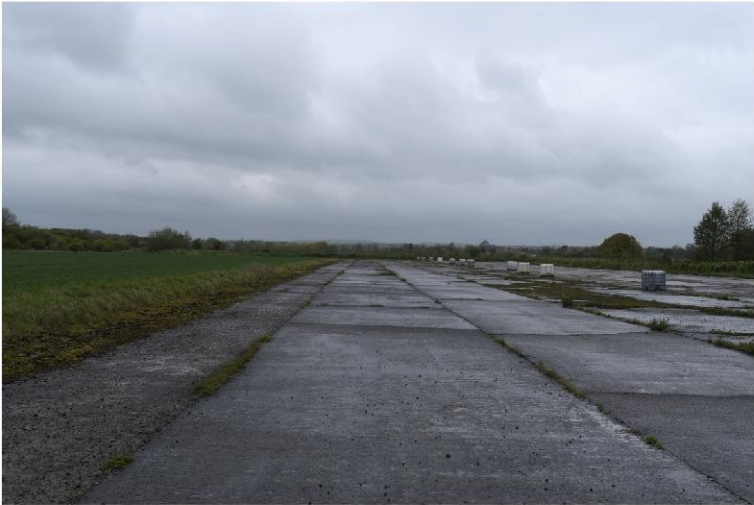
Runway 17/35 looking north (17 end)
